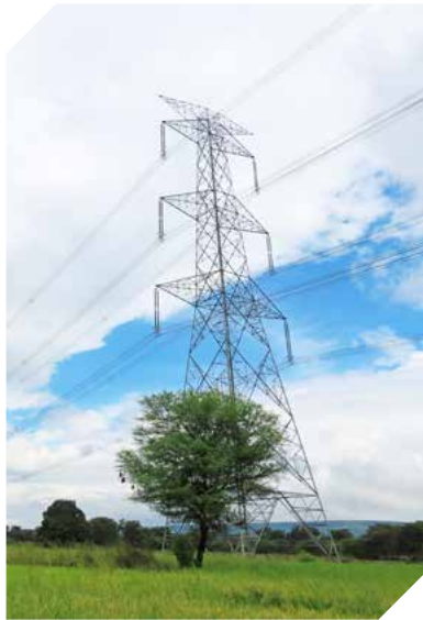
Jabalpur Power Transmission Ltd
