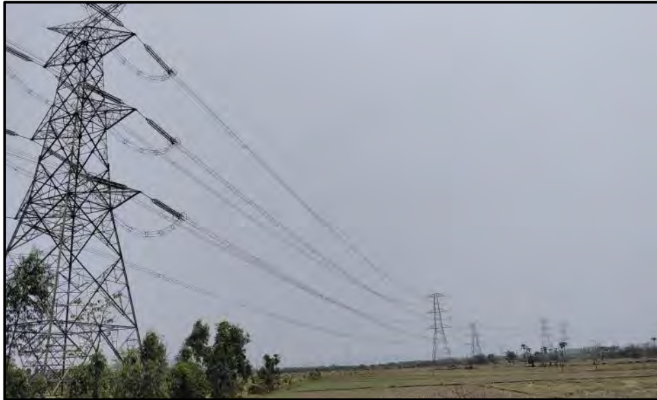
Angle Tower of 765 kV Transmission Line
