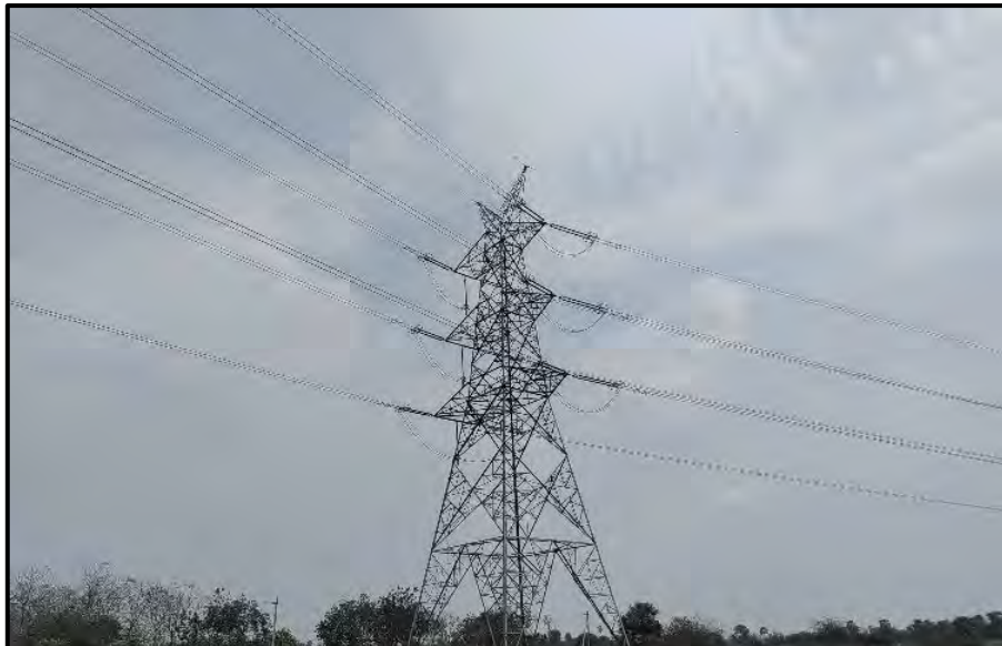
Angle Tower of 400 kV Transmission Line
