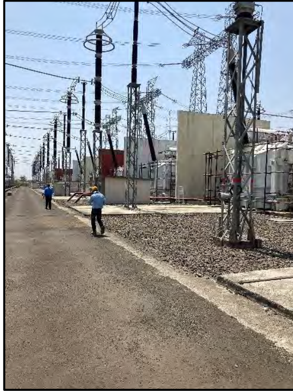
Inter Connected Transformer (ICT) – 7 x 500 MVA
