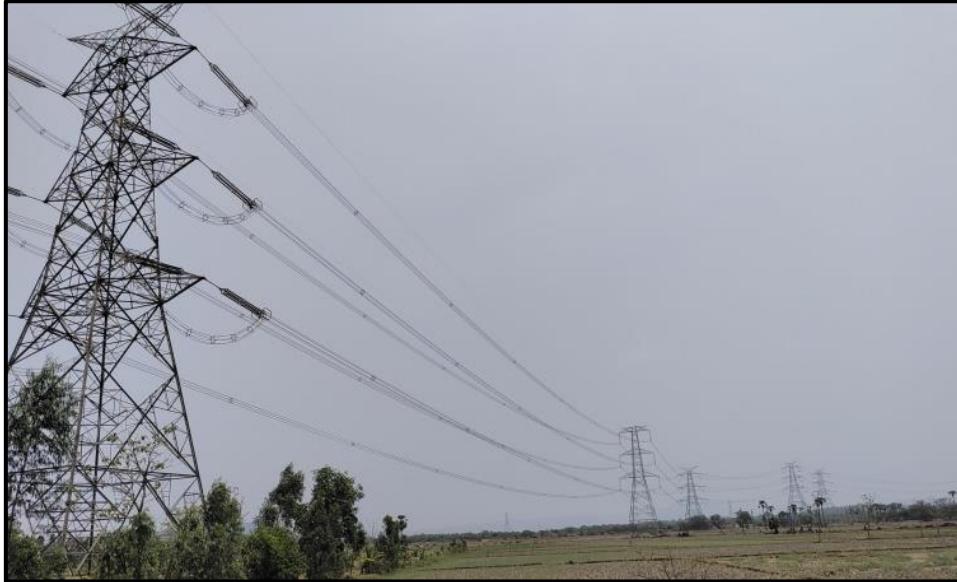
Angle Tower of 765 kV Transmission Line
