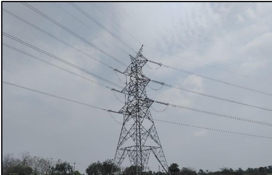
Angle Tower of 400 kV Transmission Line
